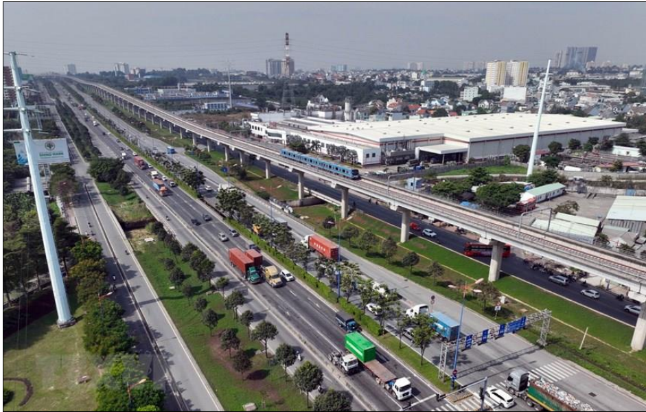
Fig 2: Railway line No. 1 (Ho Chi Minh City).
