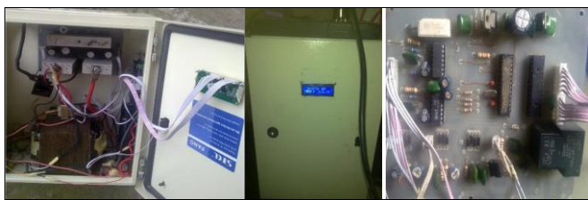
Fig 18: complete construction of 2.5kva
